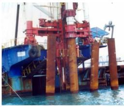
Testing a marine steel tubular pile
